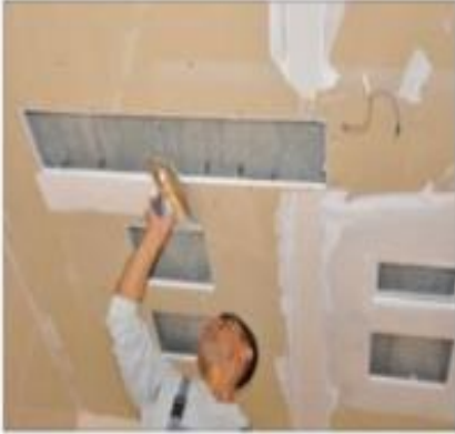
PUTTY SHOULD BE APPLIED IN TWO LAYERS AND JOINT GYPSUM SHOULD BE USED
