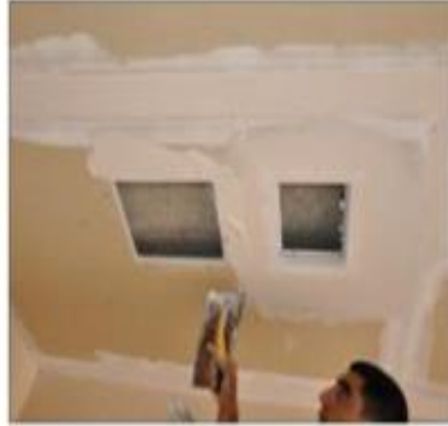
PUTTY SHOULD BE APPLIED IN TWO LAYERS AND JOINT GYPSUM SHOULD BE USED
