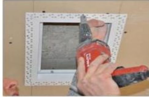
OUTER FRAME SCREWING IS MADE BY FASTENING SCREWS TO THE EXTREMITIES
