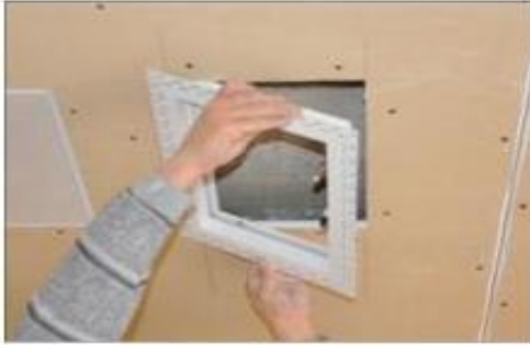
ASSEMBLY OF OUTER FRAME
