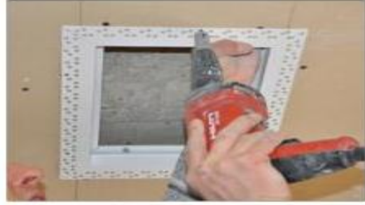
DIŞ ÇERÇEVE VIDALAMASI EN UÇLARDAN YAPILIR OUTER FRAME SCREWING IS MADE BY FASTENING SCREWS TO THE EXTREMITIES
